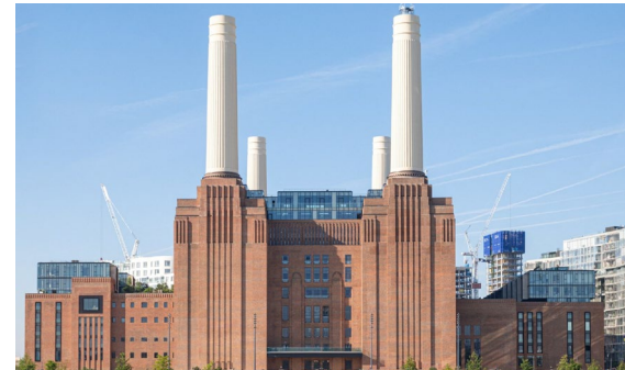
Battersea Power Station fire suppression systems
