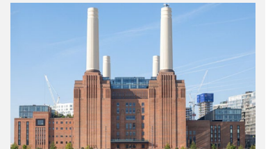
Battersea Power Station fire suppression systems
