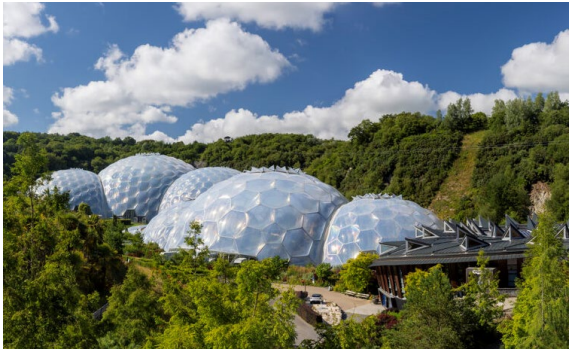
Eden Project 140 kWp roof-mounted solar PV system on plant and education facility
