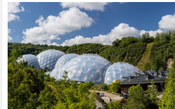
Eden Project 140kWp roof-mounted solar PV system
