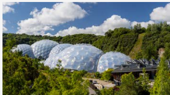
Eden Project 140kWp roof-mounted solar PV system on plant & education facility
