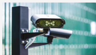
DWP upgrade of critical security infrastructure
