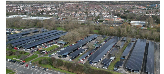
Lakeside North Harbour, UK's largest solar carport canopy
