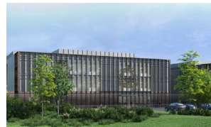
Ark, Longcross Park M&E design and build of first phase of new data centre
